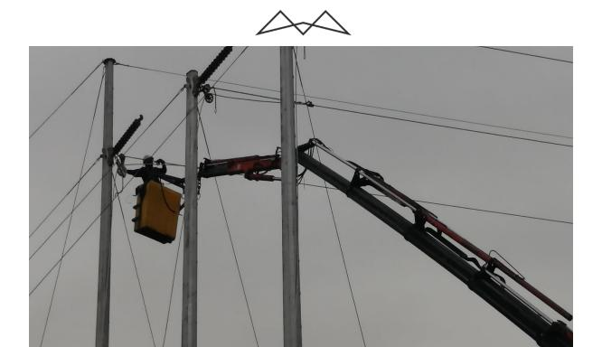
Figure 5: Tensioning of the electrical cables.
